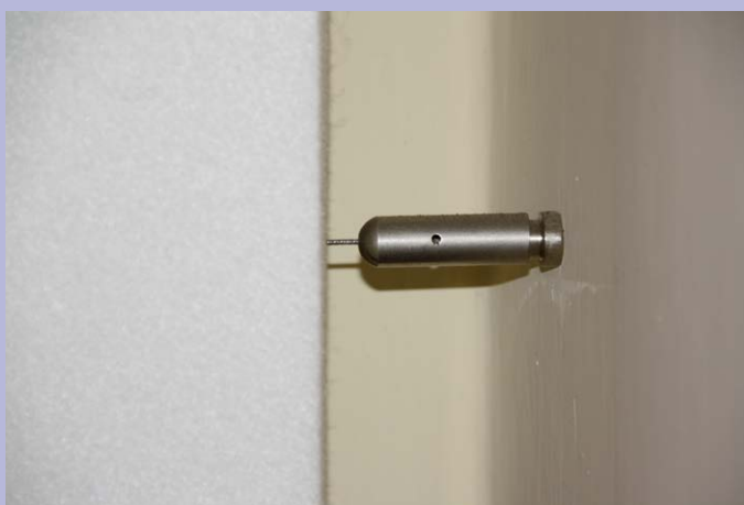
Fixing systems of panels' support cables
